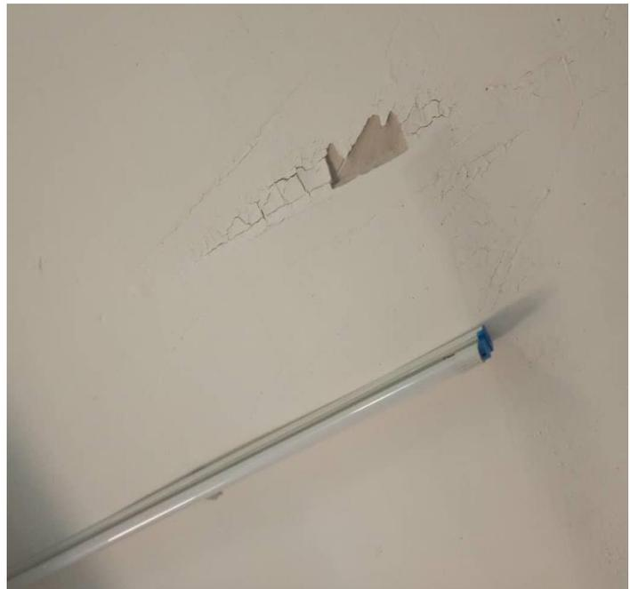
Defective painting due to leakage in floor slab
