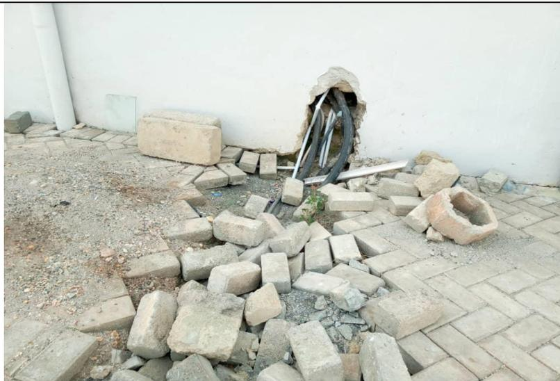
Service hole ought to be made good and paving works completed at the Library Complex
