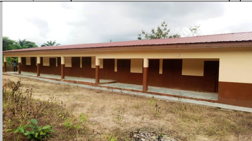
Provision of rain-gutter could to avert the splashing of rainwater to stain the surfaces of the painted walls. The conduit could be used to harvest rainwater.
